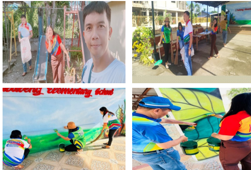
Faculty participants doing cleaning and painting work at Balaleng Elementary School
